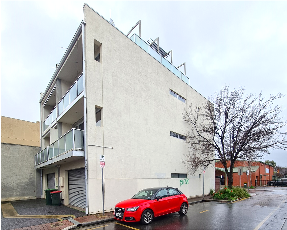
Photo 3.5 – Adjacent dwellings at 122 Gilles Street, Adelaide
