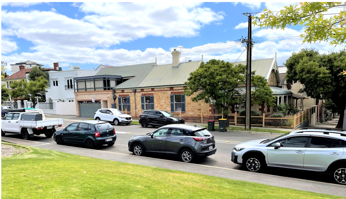
Photo 3.3: View of subject site looking northeast
