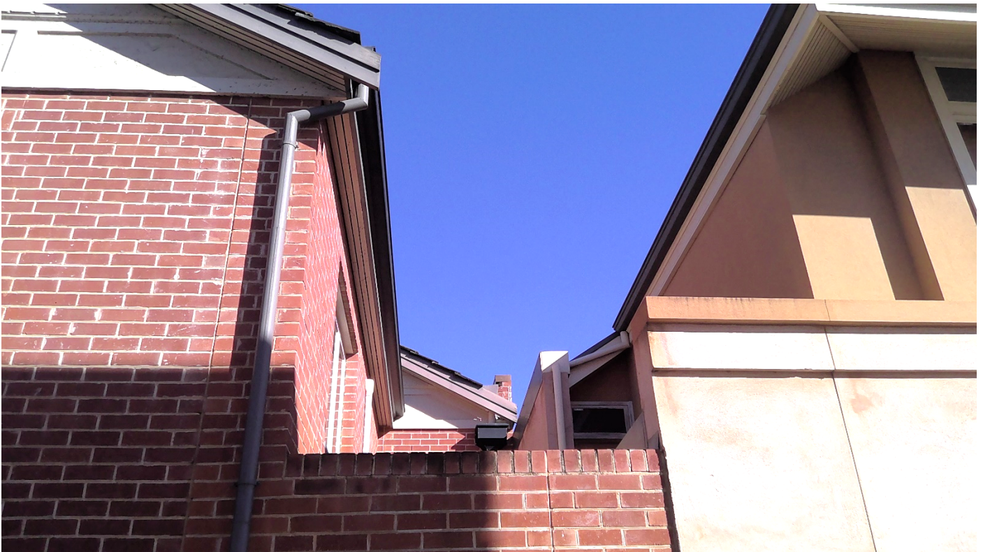
Photo 3.8: Current separation to the rear between 156 and 158 Kermode Street
