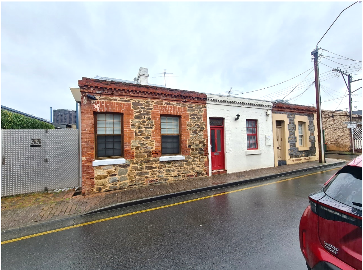
Photo 3.6 – Dwellings directly north of the subject site on Stephens Street
