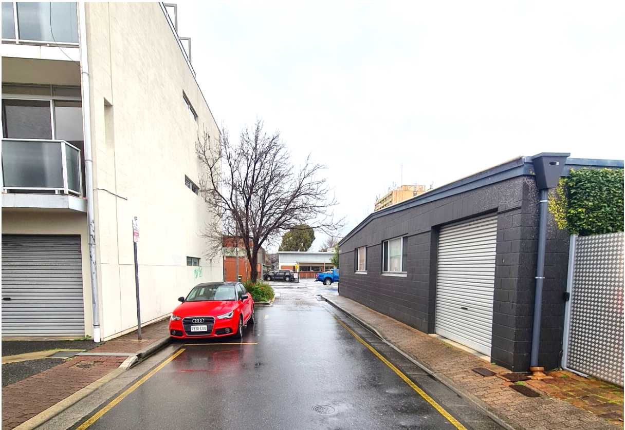
Photo 3.4 – Stephens Street looking south with subject site to the right
